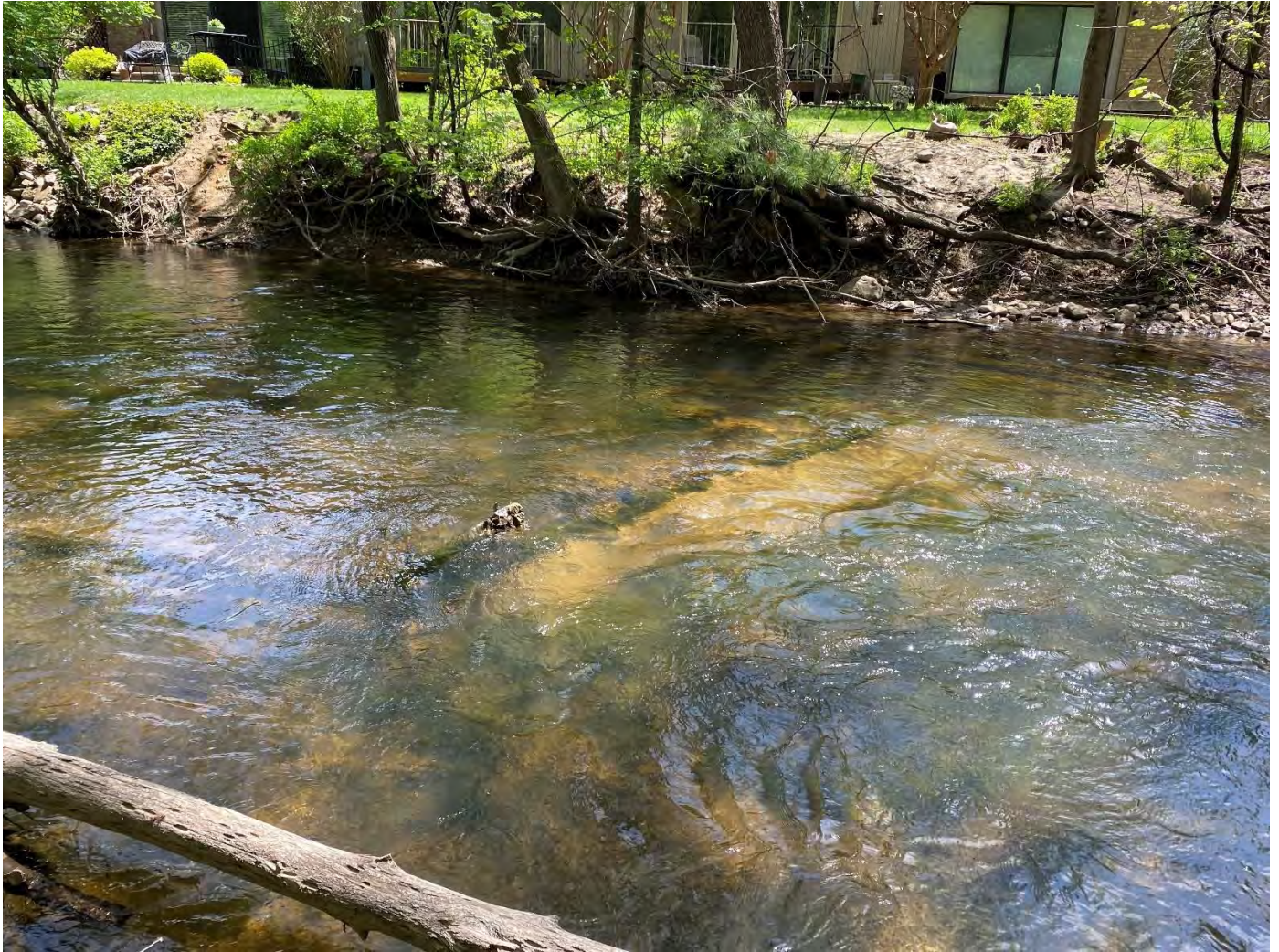
Habitat Structure 7 – A log structure was installed across the stream flow to provide cover and riffles in a slow flow area. Note the deeper pool that has formed downstream of the log.
