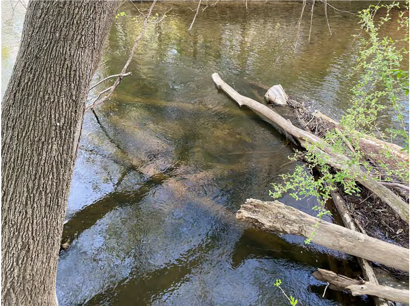
Habitat Structure 8 – Another view of the logs placed in the deeper pool to protect the bank and to provide in-stream habitat.
