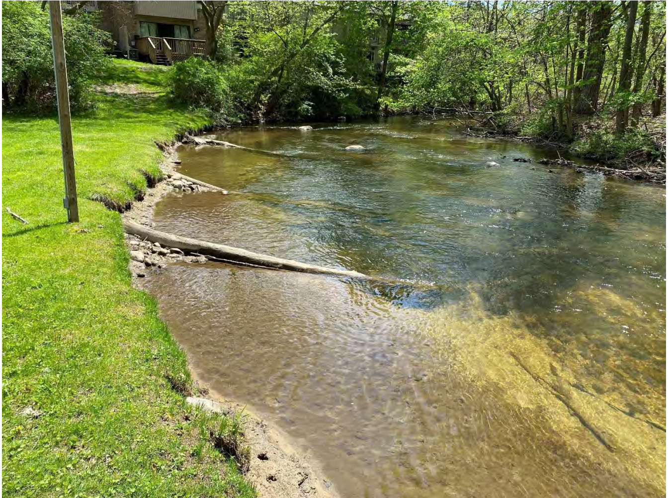
Habitat Structure 4 – Three vanes were placed in a high erosion area to build up the bank and to create more stream center flow. You can see the silt & sand buildup along the bank they are creating.
