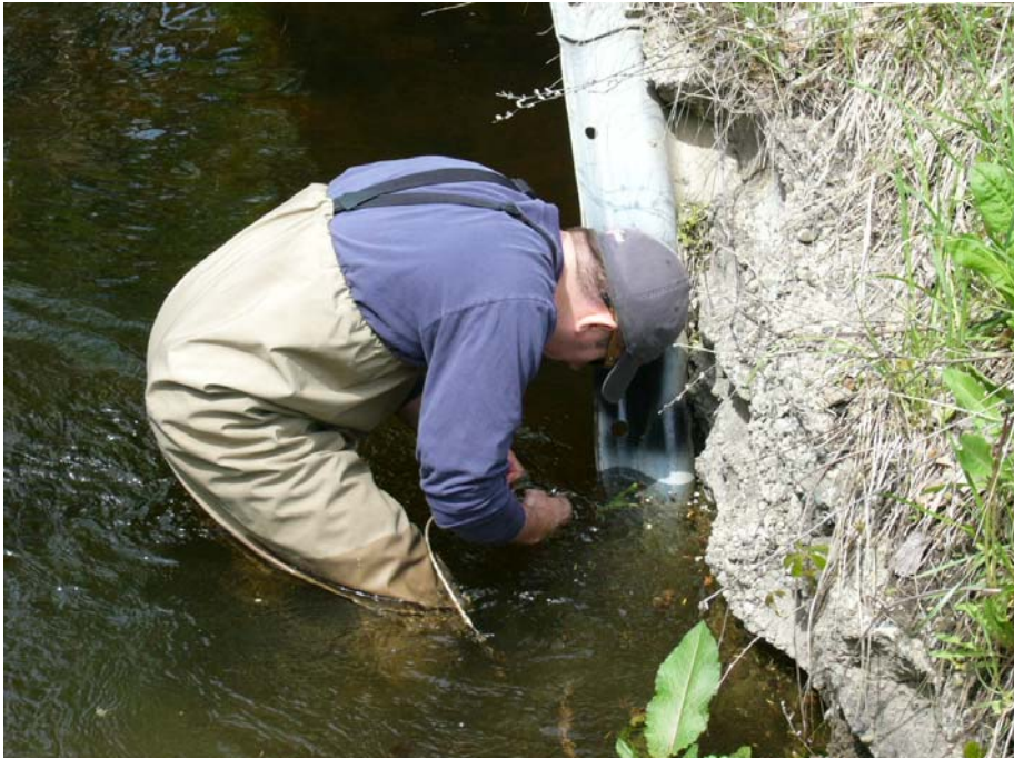
Jeff Aisthorpe of the Clinton Valley Chapter installs a temperature monitor at Atwater Bridge.
